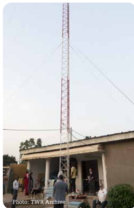
Left: The offices and transmitting tower in Yamoussoukro.
